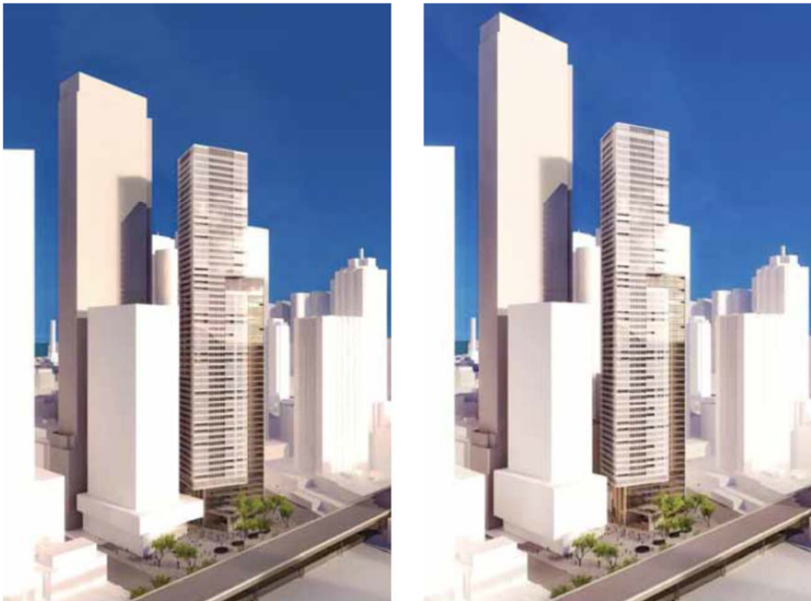
Figure 6: Tower A envelope with 900mm eastern extension (left) v. Tower A envelope as approved by D/2015/1049 (right) (Source: Urbis)
